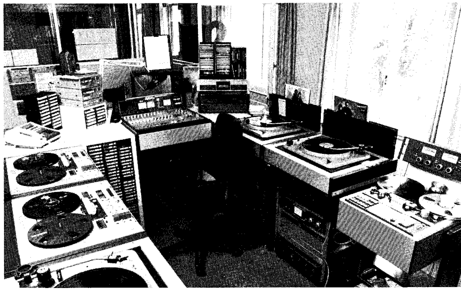
Fig. 4: The Rediffusion cable radio station
